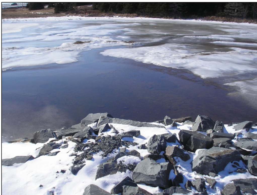
Figure 5 Central panne at LT from the culvert.
